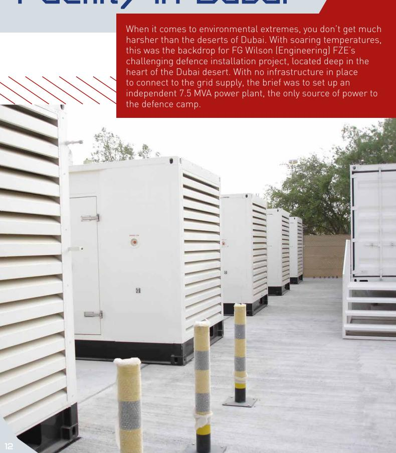
Short listed as the specialist supplier of power solutions, FG Wilson (Engineering) FZE provided a complete turnkey package consisting of five x P1500P3 containerised generator sets. The complete pre-sales engineering including selection of switchgear, synchronising controls, fuel system, yard lighting, earthing etc was carried out by a specialist application engineering team, supported by the FG Wilson Power Solutions team.
